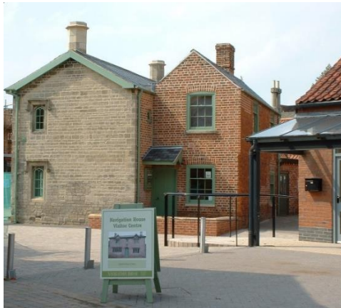
Wheelchair access via the side door.
